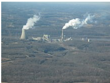
Zimmer power plant
