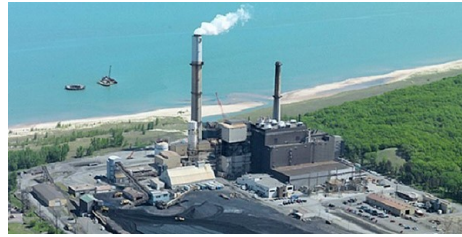
Bailly Generating Station
